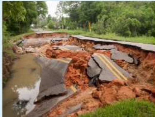
Flooding of a small stream in June 2014 destroyed this roadbed in Foley. Credit: Patsy Lynch, FEMA.
